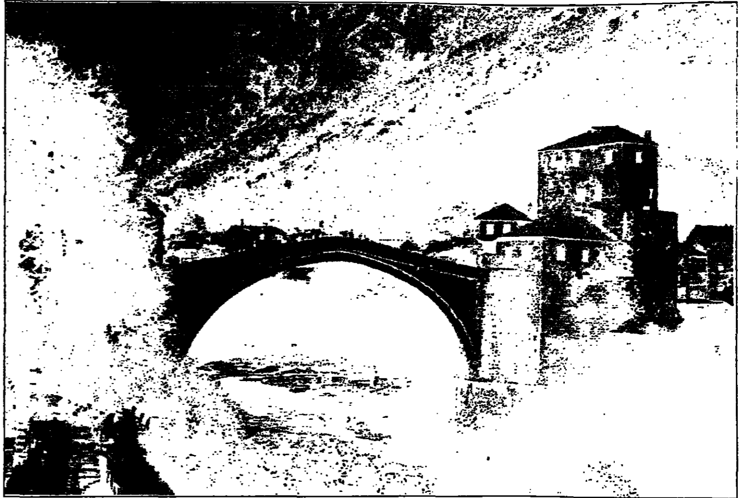
This negative print of a stone bridge from a color slide produces an interesting effect since the colors "filter" the light passing through at different intensities.
